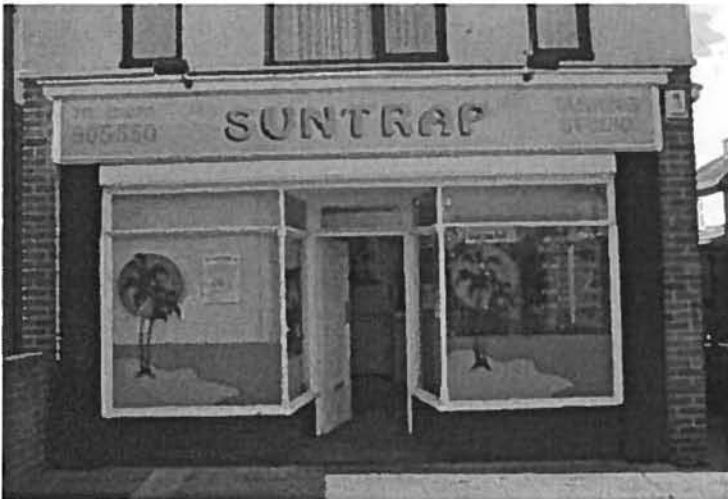
The amount of signage on these windows exceeds the 20% allowed to cover the windows
