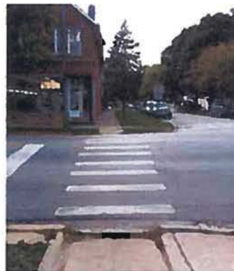
Highly visible crosswalks are appropriate at intersections with heavy pedestrian activity.
