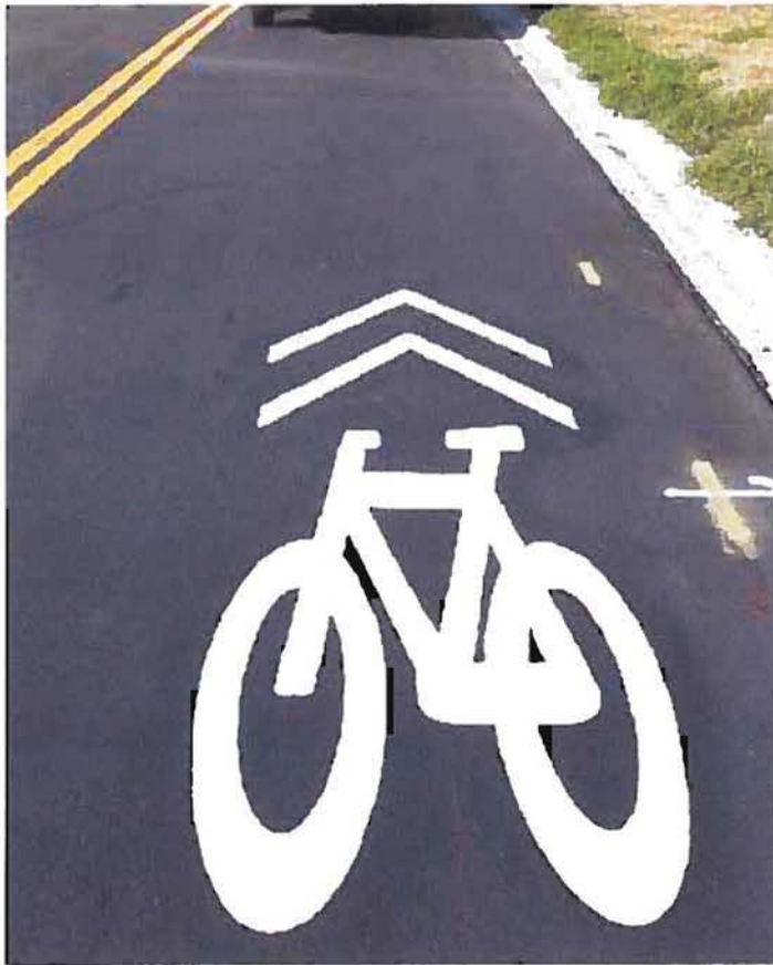
Shared lane markings on roads may help increase driver awareness of students who bike to school.
