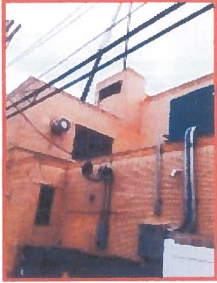
The Tower Requires Brick Replacement at the Vent, Cut Control Joint, and Complete with Tuck Pointing.
