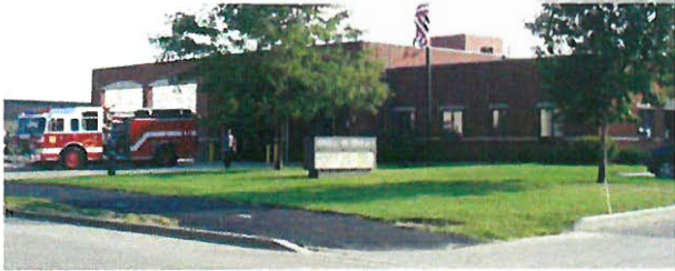
Village of Romeoville Fire Station Addition Project Value: $1.1M | Design-Build
