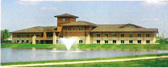
Village of Elwood Police Station and Municipal Center Project Value: $7.8M | Design-Build
